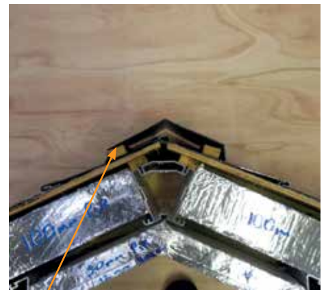
24. Fix timber batten on for ridge & hip.
