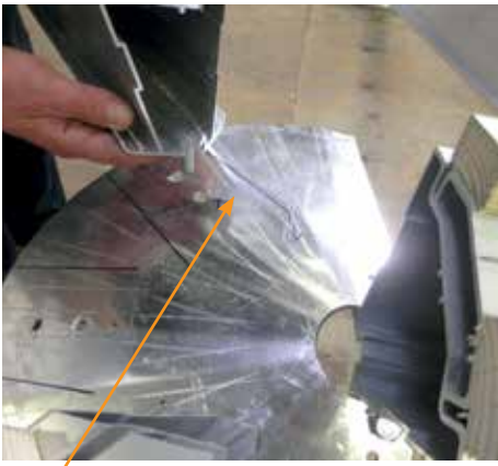
10. Secure Hips into Ridge End Plate using 13mm bolts supplied.
