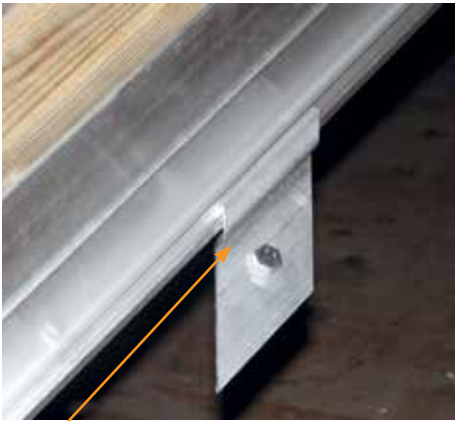
13. A typical jack rafter kit in place
